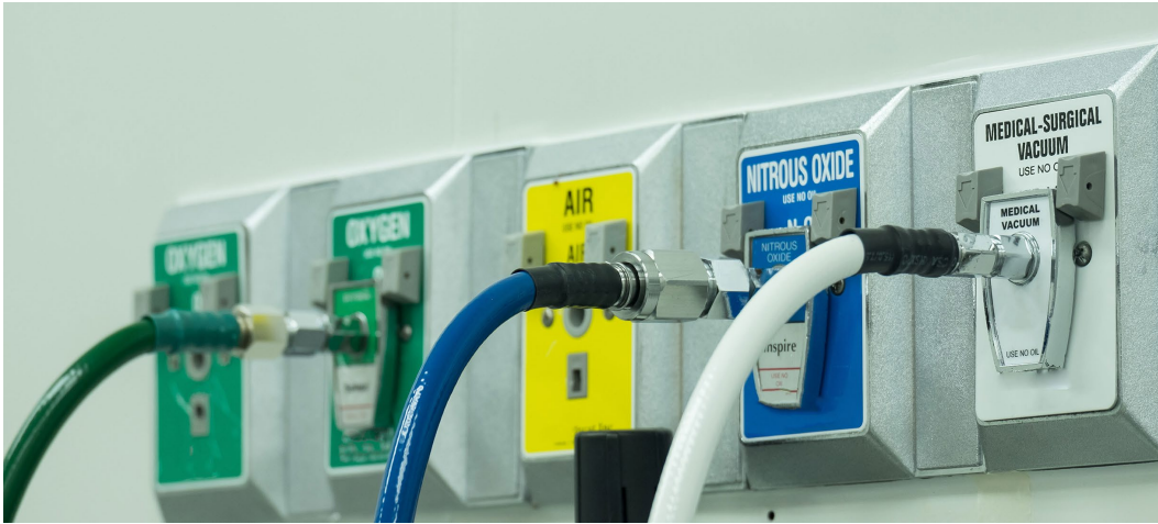
Medical gas lines are usually designed to handle 150% of average usage, not the unprecedented surge from increased ventilator use during the COVID-19 pandemic.
